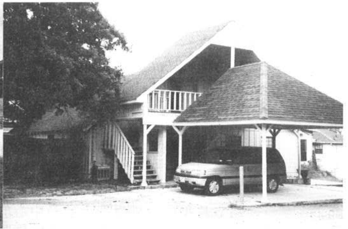
行政樓 Administration Building
